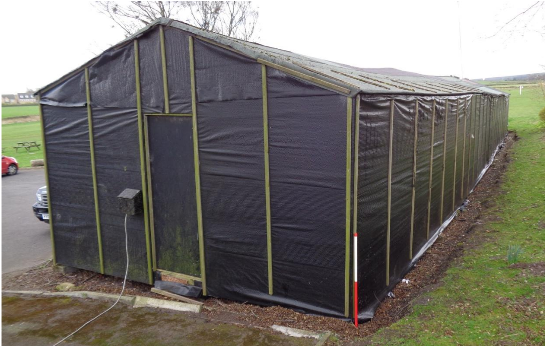
An Accommodation Hut at Redmires, Sheffield. Note the use of a ranging pole for scale.
