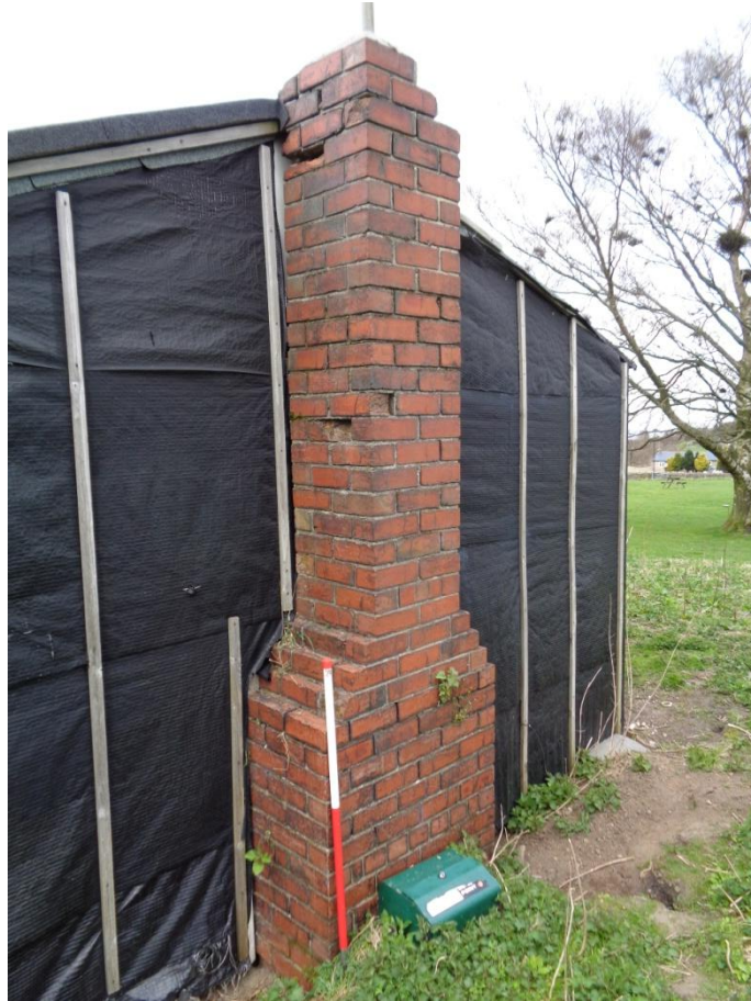
A photograph highlighting a feature of the Accommodation Hut at Redmires, Sheffield.
